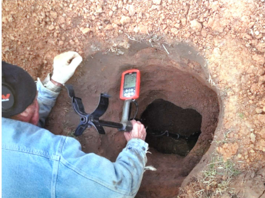
Figure 5 - Second dig at same site with a deeper and wider hole
